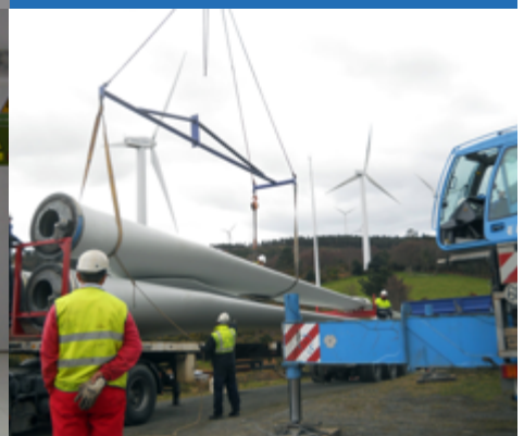
Assembly and disassembly of blades and rotors
